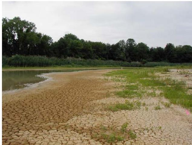
Figure 4. Desiccation cracks in Pond 1 area looking toward slurry pond dike.
